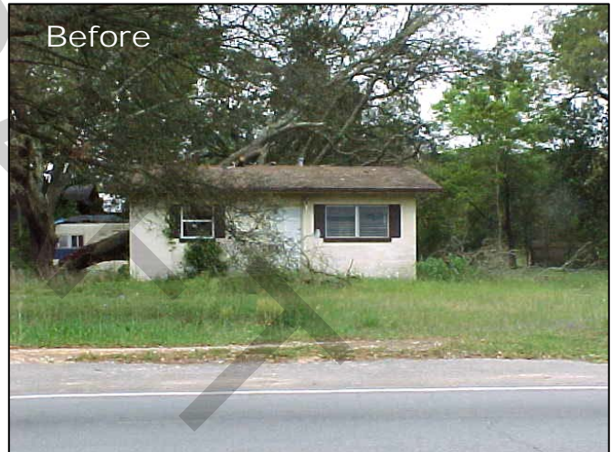
The dilapidated structure shown above (bottom image) was demolished during Q2 FY2015.
