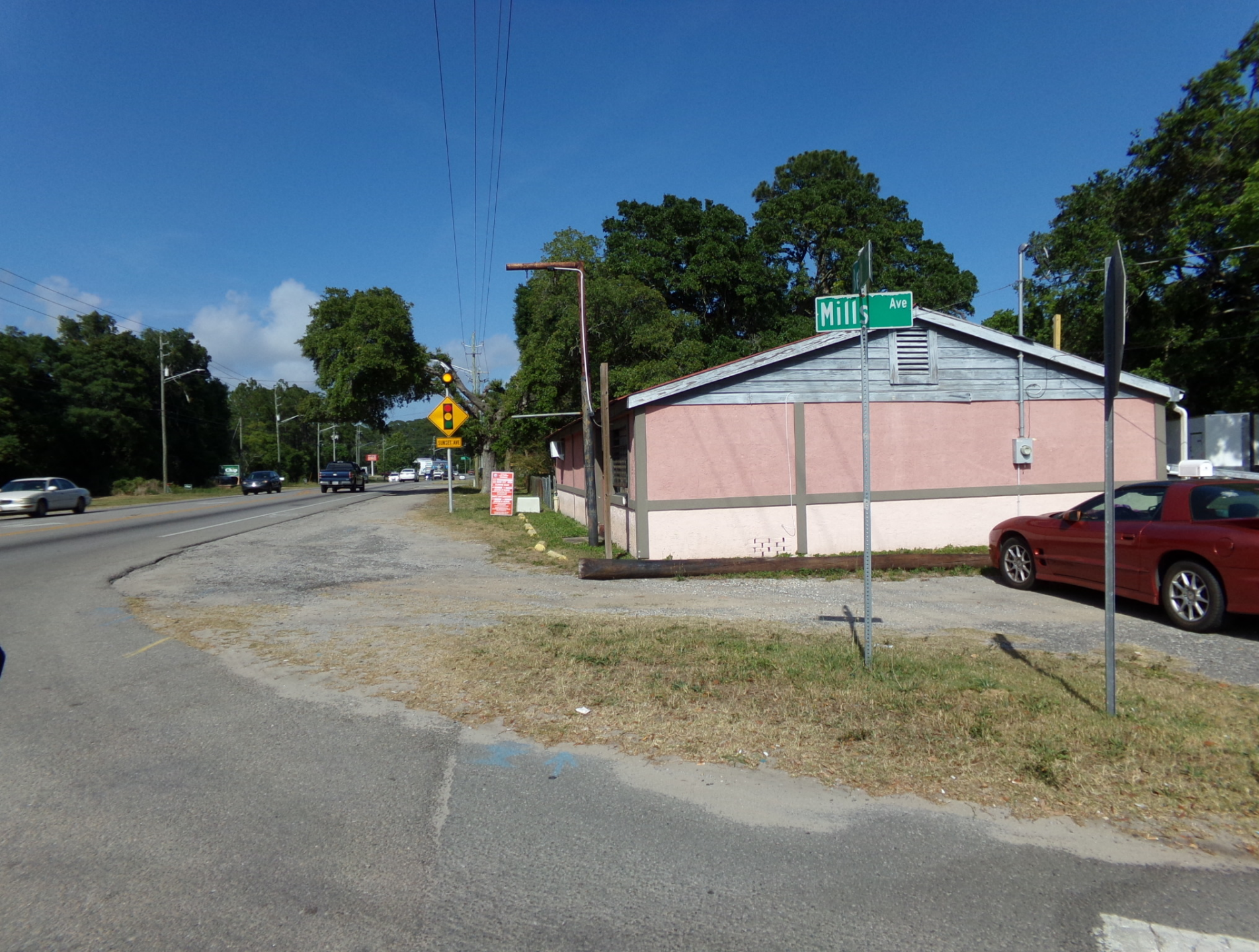
Another view of subject property, looking east
