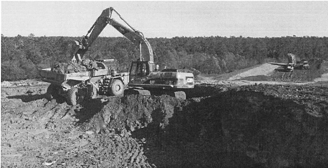
Figure 3-1. Final Cover Soil Excavation and Transportation
