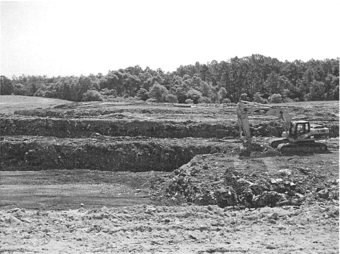
Figure 3-6. Benches Resulting from Excavation Operation
