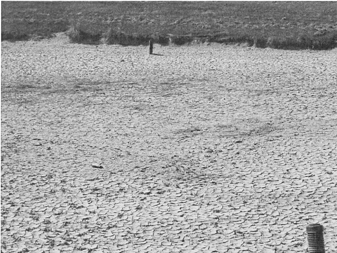
Figure 3-16. Clay/Silt Layer Build-up in the Stormwater Pond
