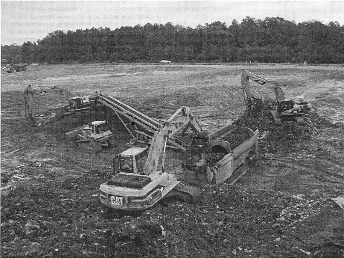
Figure 3-7. Relative Positions of Various Equipment during Track-Mounted Screen Use
