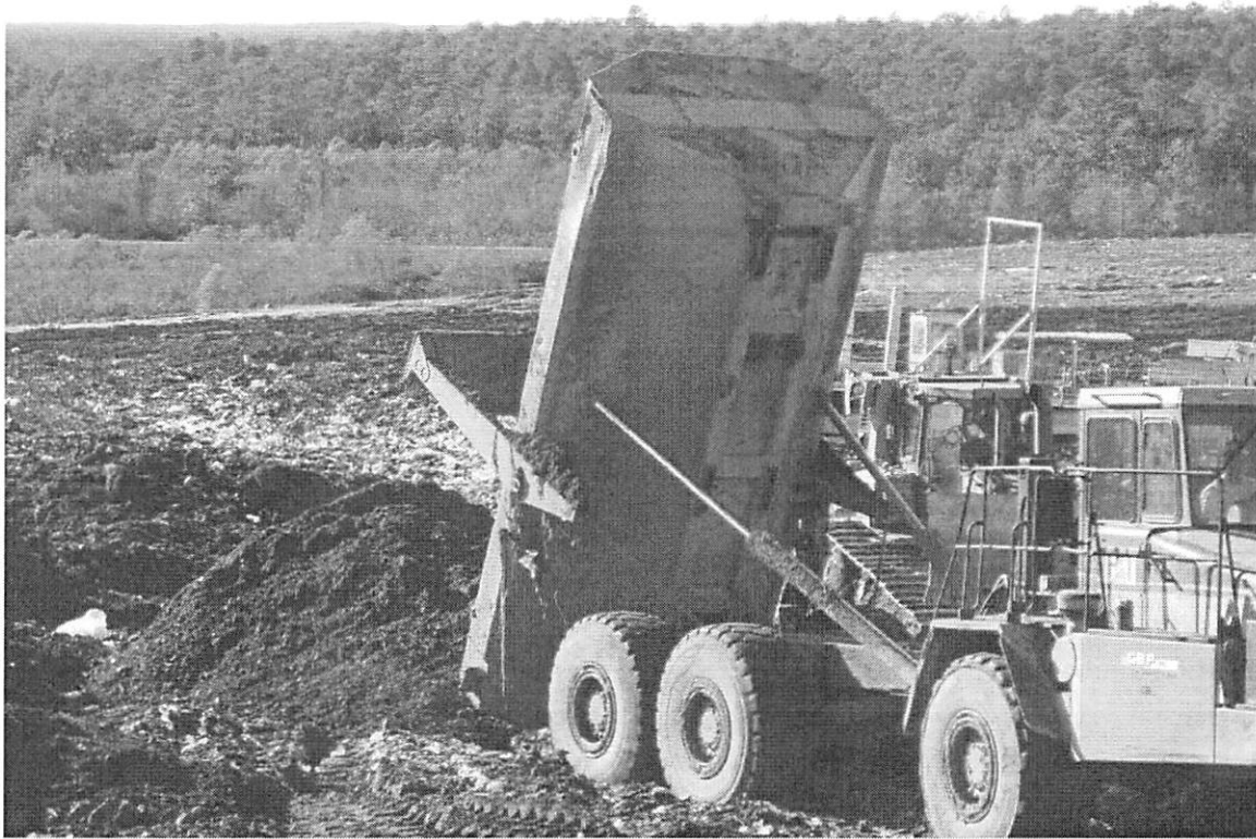
Figure 3-10. Stockpiling of Reclaimed Soil Near the Active Working Face for Use as Daily Cover
