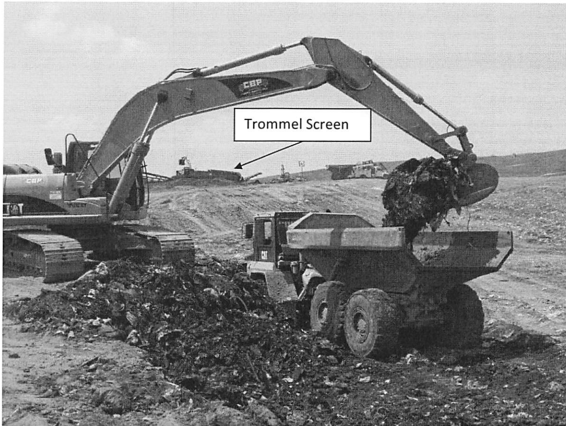
Figure 3-3. Waste Excavation and Transportation Operation
