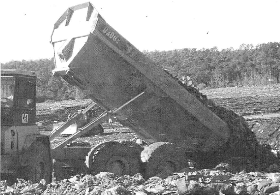
Figure 3-9. Unloading of Screened Waste at the Active Disposal Area
