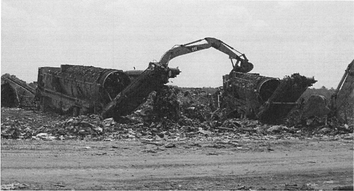
Figure 3-5. Loading of the Excavated Waste onto Screens
