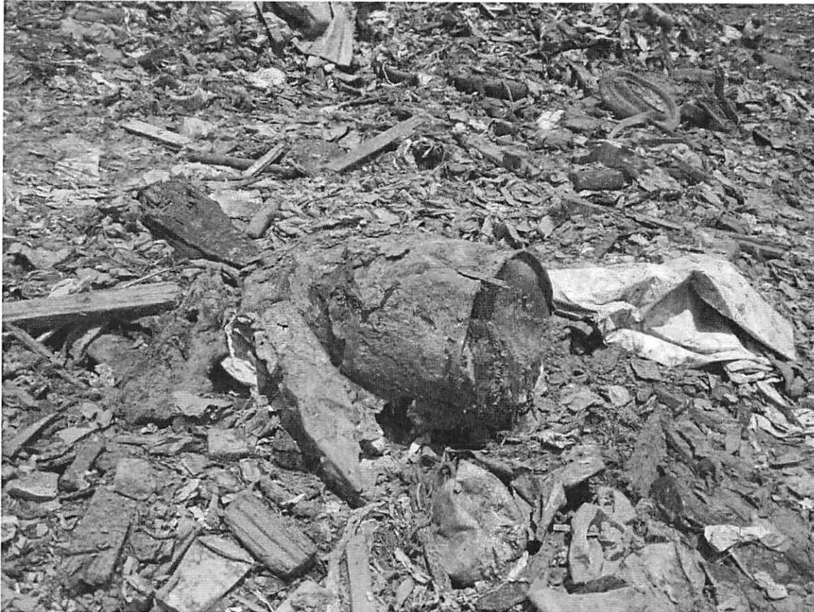
Figure 3-13. A Picture of a Drum Encountered During the Waste Excavation Process
