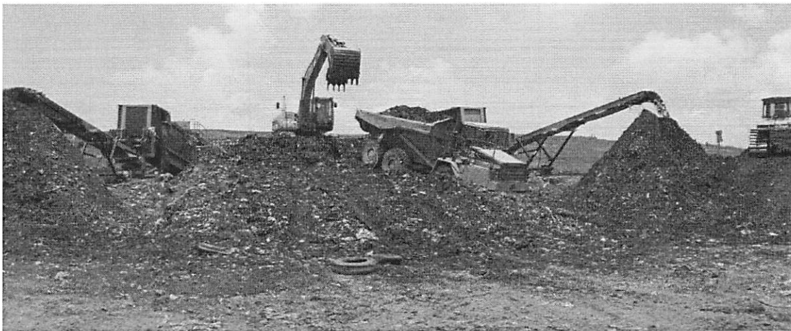
Figure 3-4. Stockpiling of the Excavated Waste between the Screens
