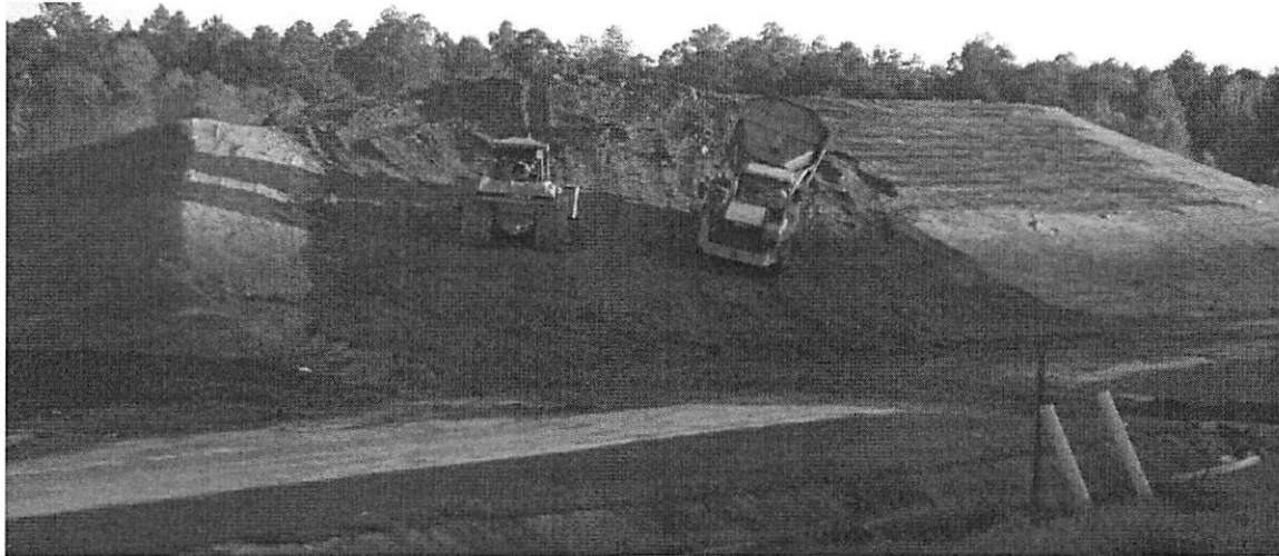
Figure 3-2. Final Cover Soil Stockpile
