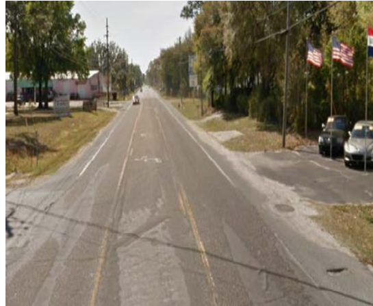
EXISTING CONDITION: E. OLIVE ROAD. CRA STAFF
