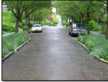
Curb Extensions with infiltration (rain gardens)
