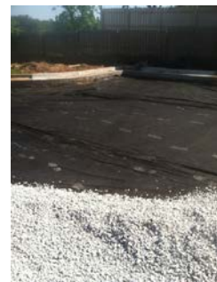
Curing the pervious concrete
