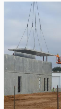
First Flat Slab (First Level, Corridor Between Area A and C)
