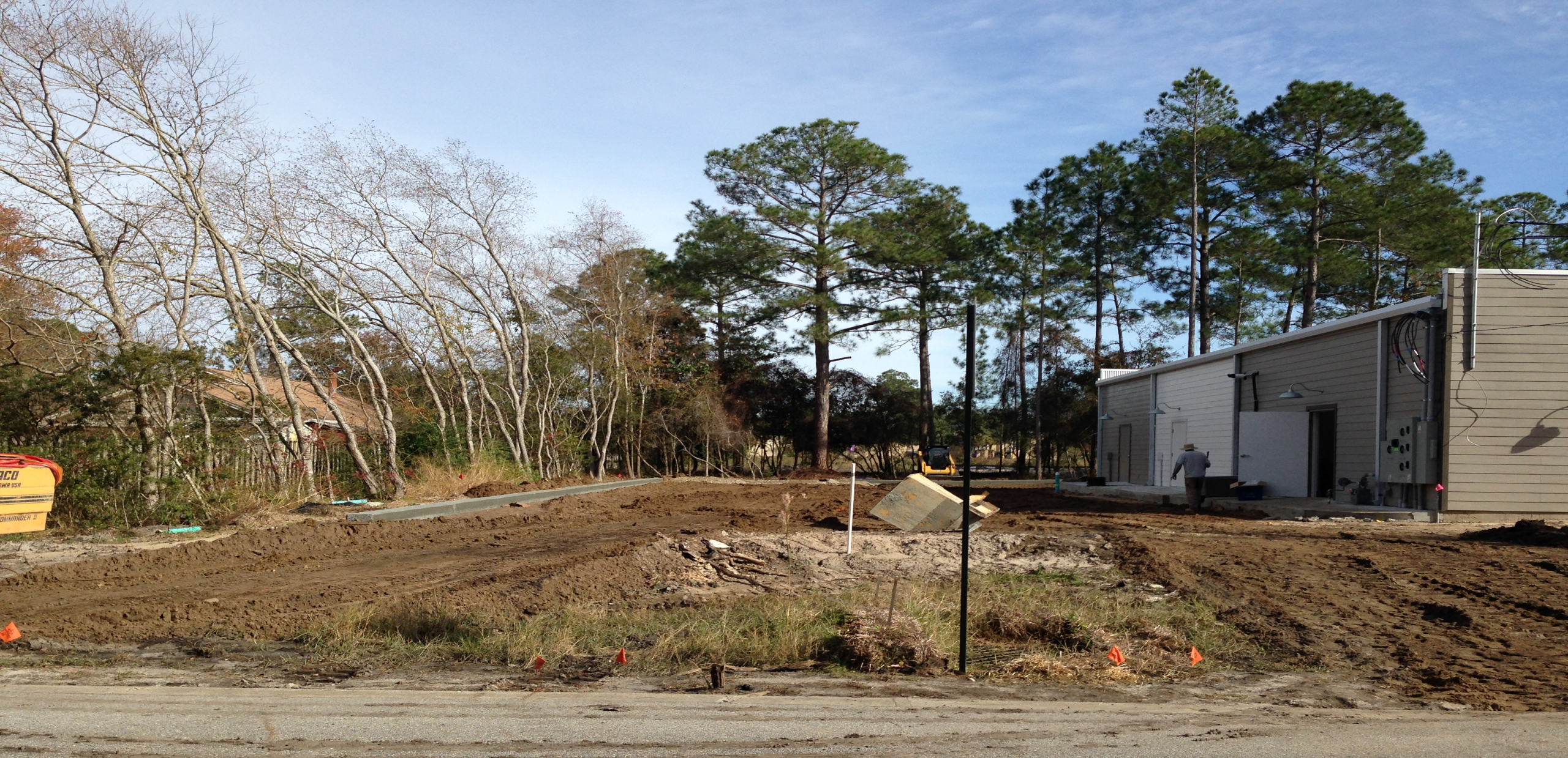
Looking East across rear of site
