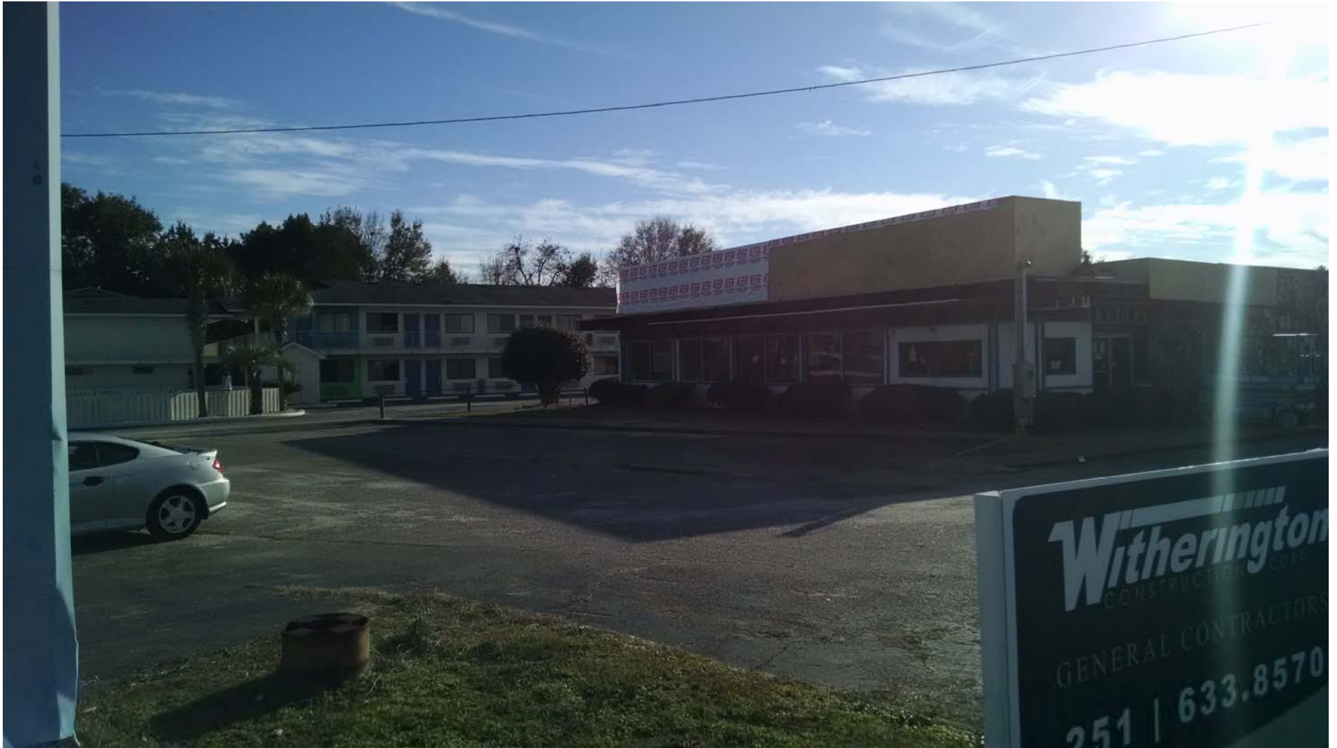
Looking West onto site
