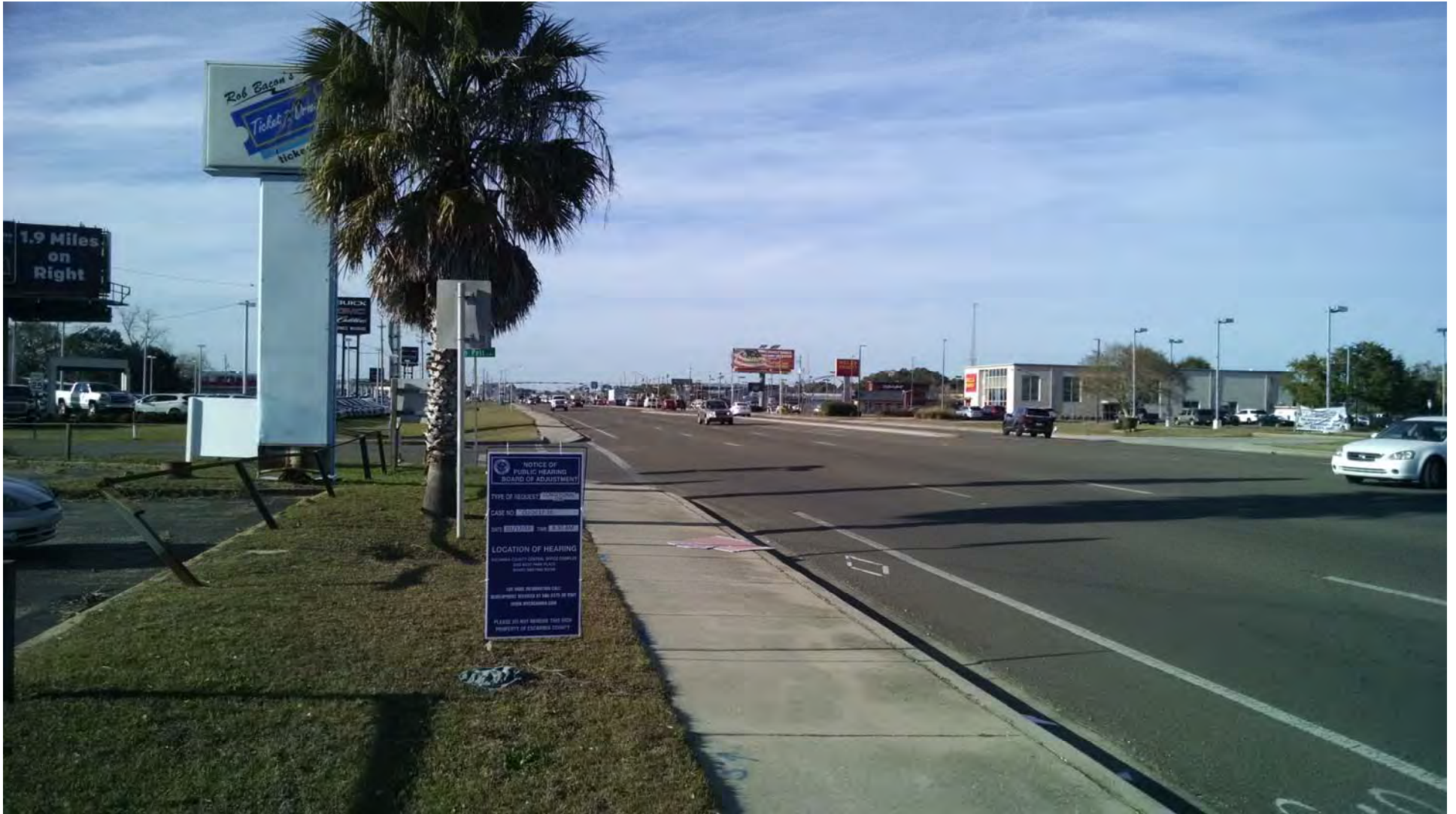
Looking North along Pensacola Blvd
