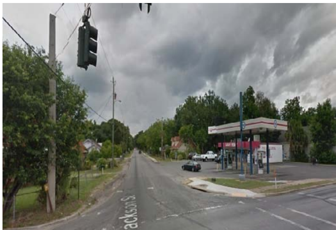
EXISTING CONDITION: WEST JACKSON STREET, GOOGLE MAPS
