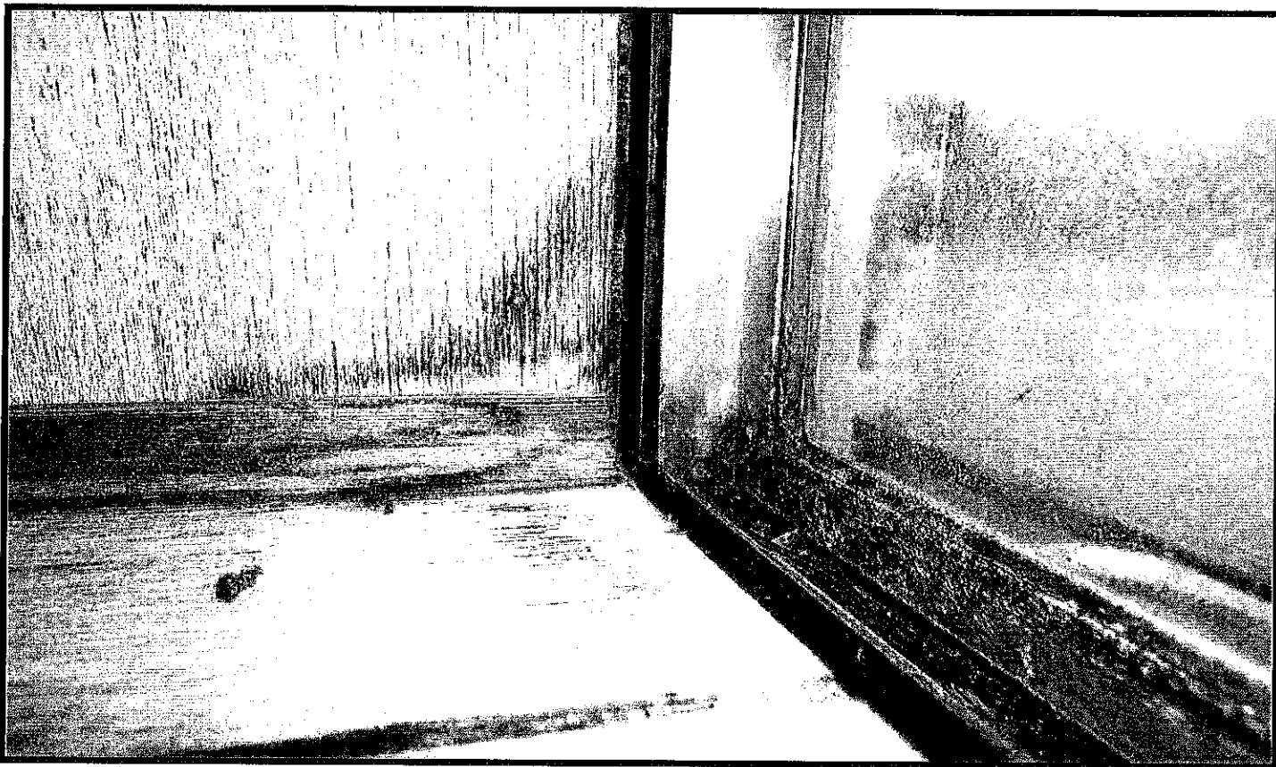
Photo No. 12: VIEW OF WATER DAMAGE OF WINDOW AREA IN THE OFFICER'S BUNK ROOM.
