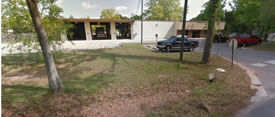
EXAMPLE OF A LIGHT INDUSTRIAL BUSINESS ON W. OAKFIELD ROAD, PHOTO: GOOGLE MAPS
