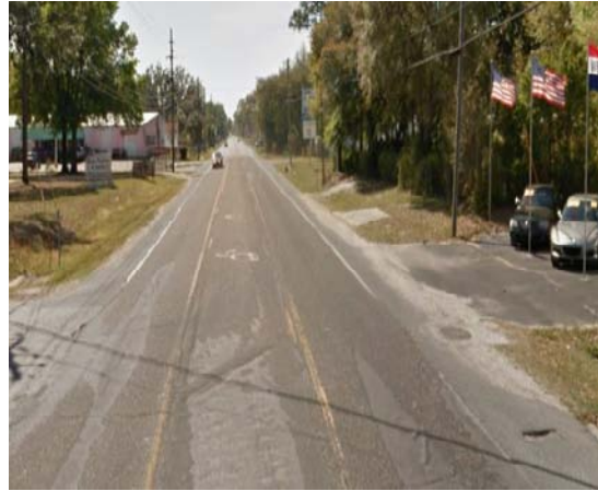
EXISTING CONDITION: E. OLIVE ROAD. CRA STAFF
