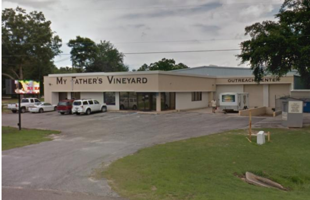
INSTITUTIONAL USES, ENSLEY CRA. PHOTO CREDIT: GOOGLE MAPS
