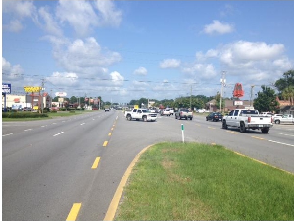
EXISTING CONDITION: E. NINE MILE RD., CRA STAFF PHOTO
