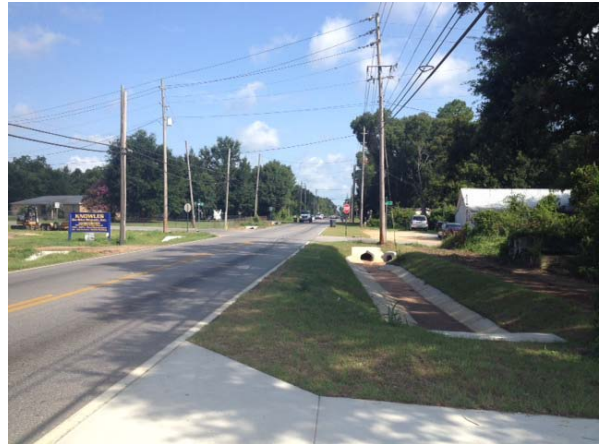
EXISTING CONDITION: N. PALAFOX STREET, CRA STAFF PHOTO
