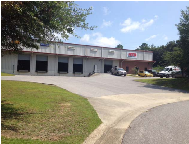
EXAMPLE OF A LIGHT INDUSTRIAL BUSINESS ON SEARS BLVD. IN ENSLEY. PHOTO CREDIT: CRA STAFF
