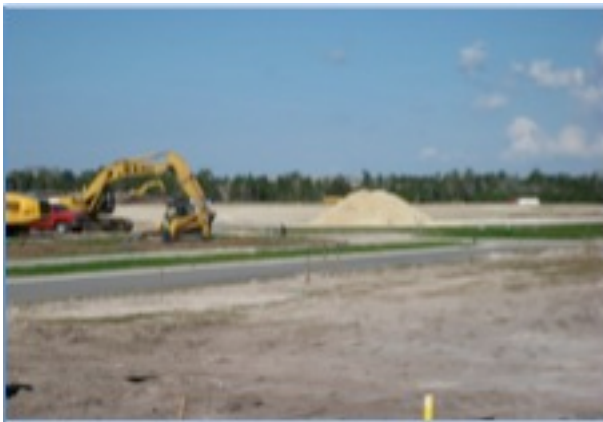
Avoid complete site clearing
