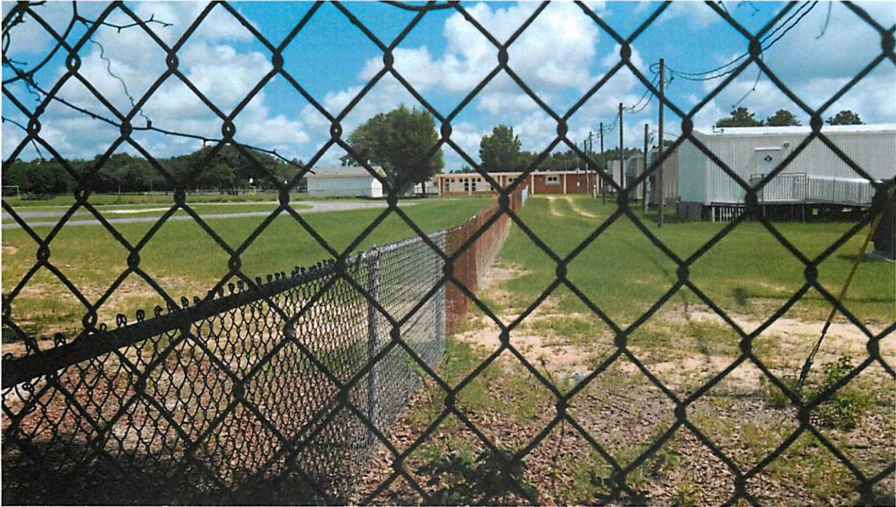
Figure 5: Rear of Parcel, facing school track and classrooms
