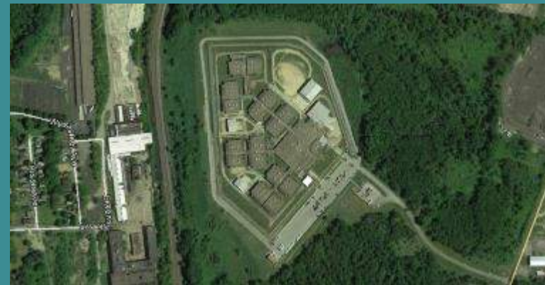
Northeast Ohio Correctional Center
