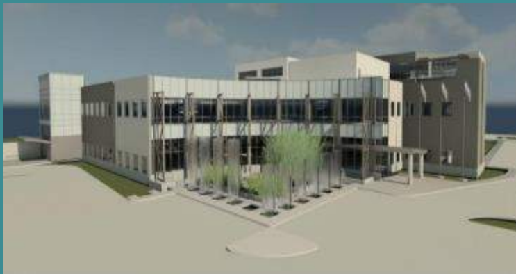
San Mateo Maple Street Jail
