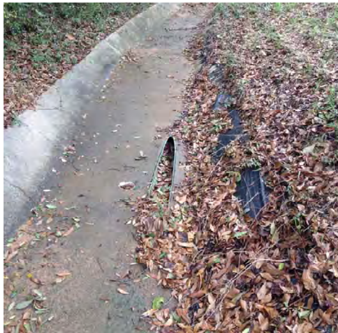
Underdrain Outfall in Ditch Along CR 97
