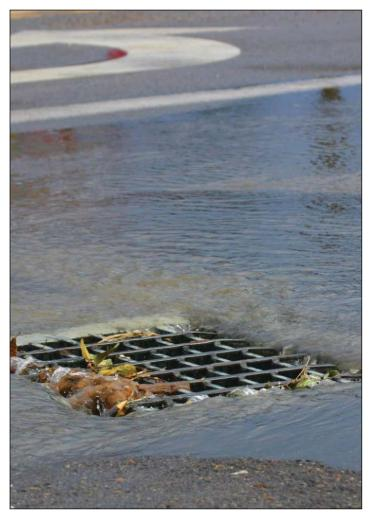
All of this stormwater entered the public infrastructure system which was also overwhelmed in many areas. Throughout Escambia County, stormwater overtopped roads where culverts and stormwater collection systems lacked the capacity to carry the historic runoff. The stresses involved in roadway overtoppings caused erosion of surrounding soils which in the most severe cases caused failure of the roadways rendering them incapable of carrying traffic.
