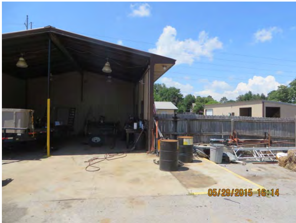
I: Northerly View of the Garage and Drums
