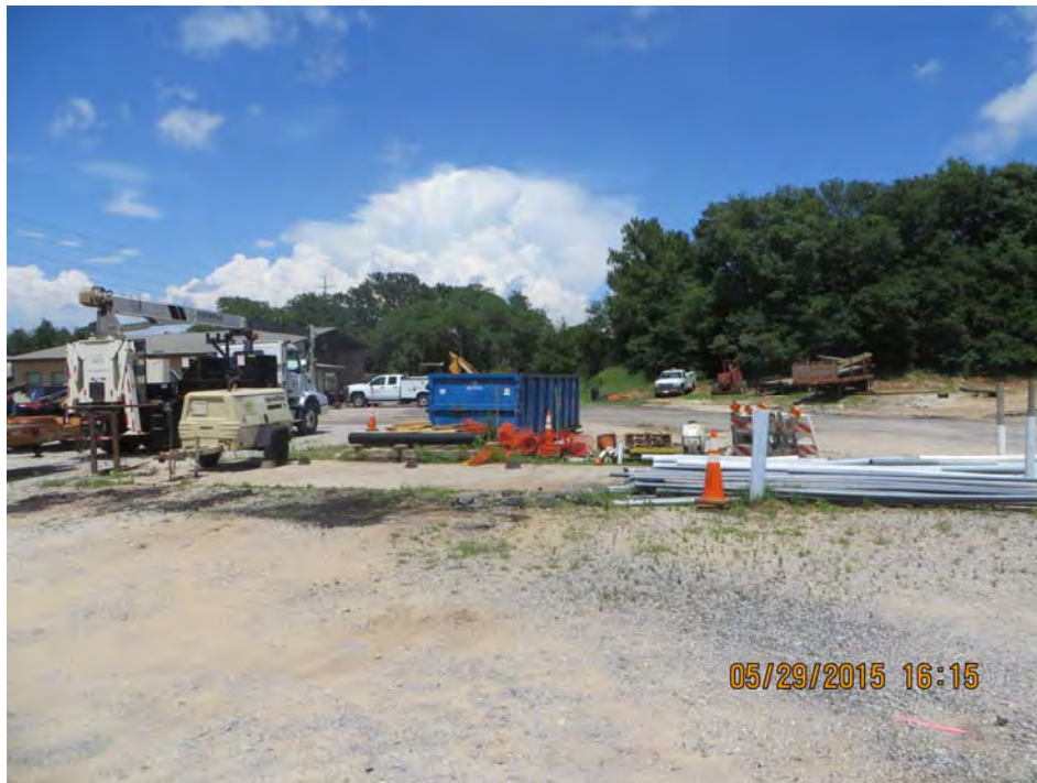
K: Easterly View of the Construction Equipment and Dumpster
