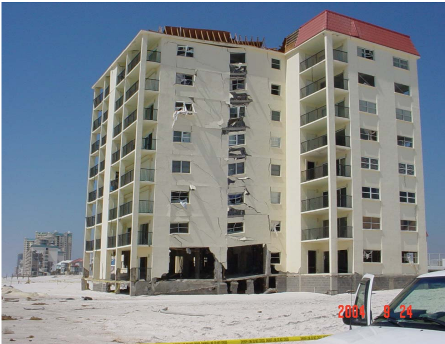
Vista Del Mar Prior to Demolition
