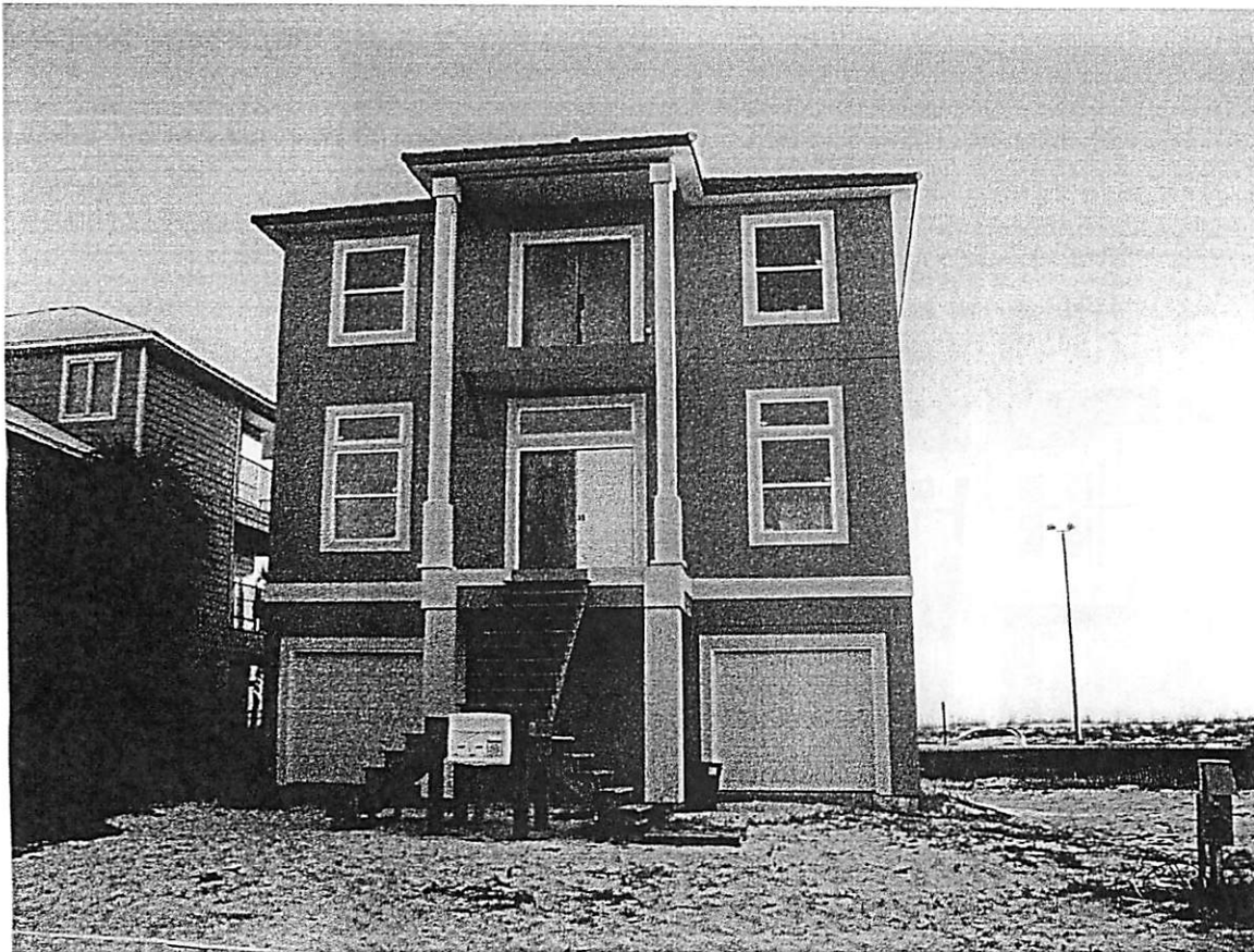
FRONT VIEW - TAKEN ON GALVEZ CT. (FACING SOUTH)
