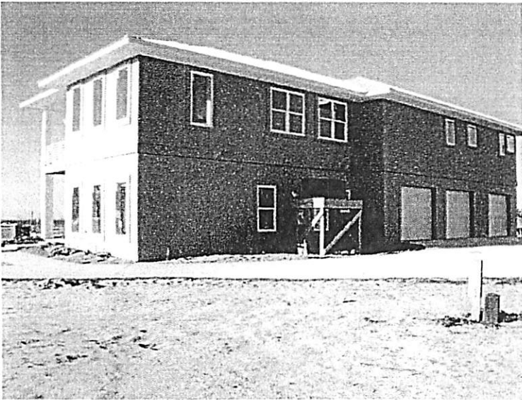
Right side view, photo taken 4-5-11
