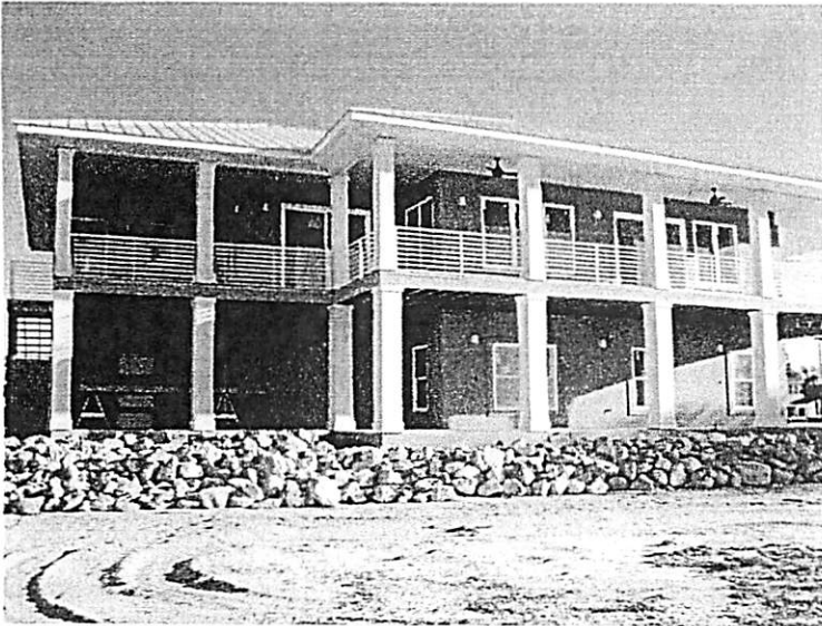
Rear view, photo taken 4-5-11
