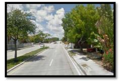
**STREETS:** Streets are local, walkable, multi-movement facilities with speeds that should be no higher than 25 mph. Streets should contain raised curbs (small corner radii, wide sidewalks, parallel parking, and trees in individual or continuous planters. The primary purpose is to serve local traffic and provide vehicular and pedestrian access to abutting properties.
