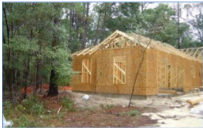
Trees were retained at this site, but avoid mounding soil around the base of the trees, as they did here!
