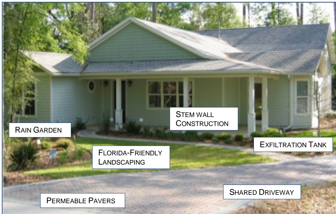
Figure 3.6. Stormwater LIDs at the Lot Scale (Medera Model Home)
