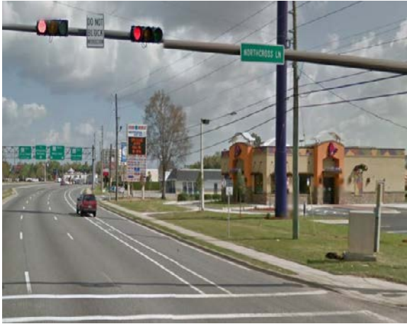
EXISTING CONDITION: N. DAVIS HIGHWAY. CRA STAFF
