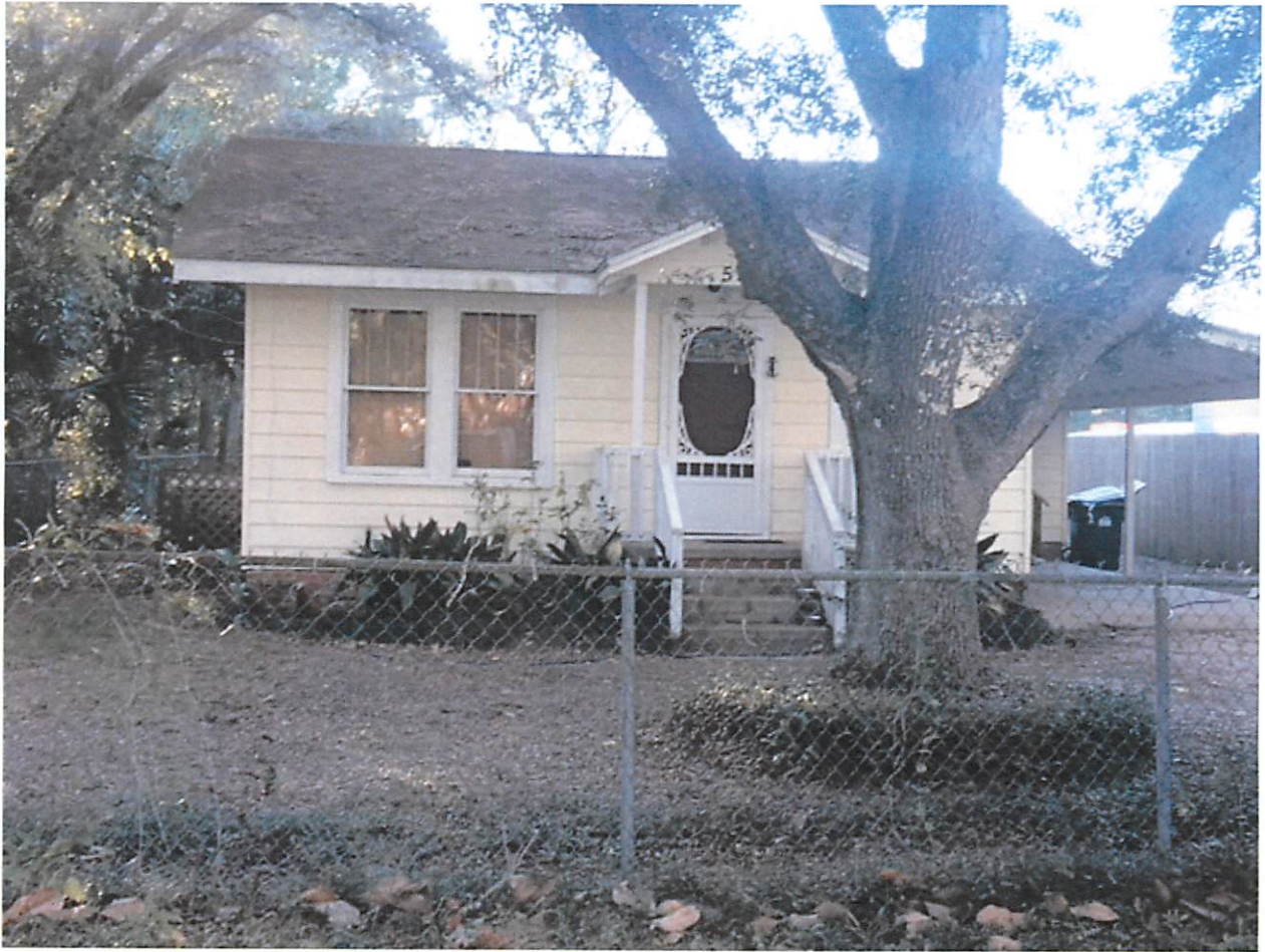
Total Electrical Rewiring Upgrade and Replacement Roof 535 South First Street – Samantha Taylor
