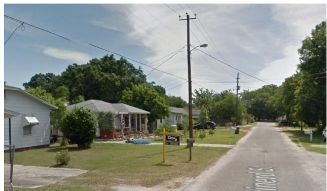
EXAMPLE OF RESIDENTIAL STREET LIGHTING, PHOTO: GOOGLE MAPS
