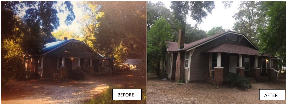
EXAMPLE OF A RESIDENTIAL REHABILITATION GRANT RECIPIENT, NEW ROOF INSTALLATION, PHOTO: CRA STAFF
