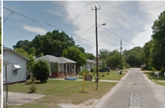
EXAMPLE OF RESIDENTIAL STREET LIGHTING, PHOTO: GOOGLE MAPS
