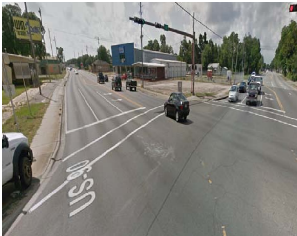
EXISTING CONDITION: -MOBILE HIGHWAY AND W STREET, GOOGLE MAPS
