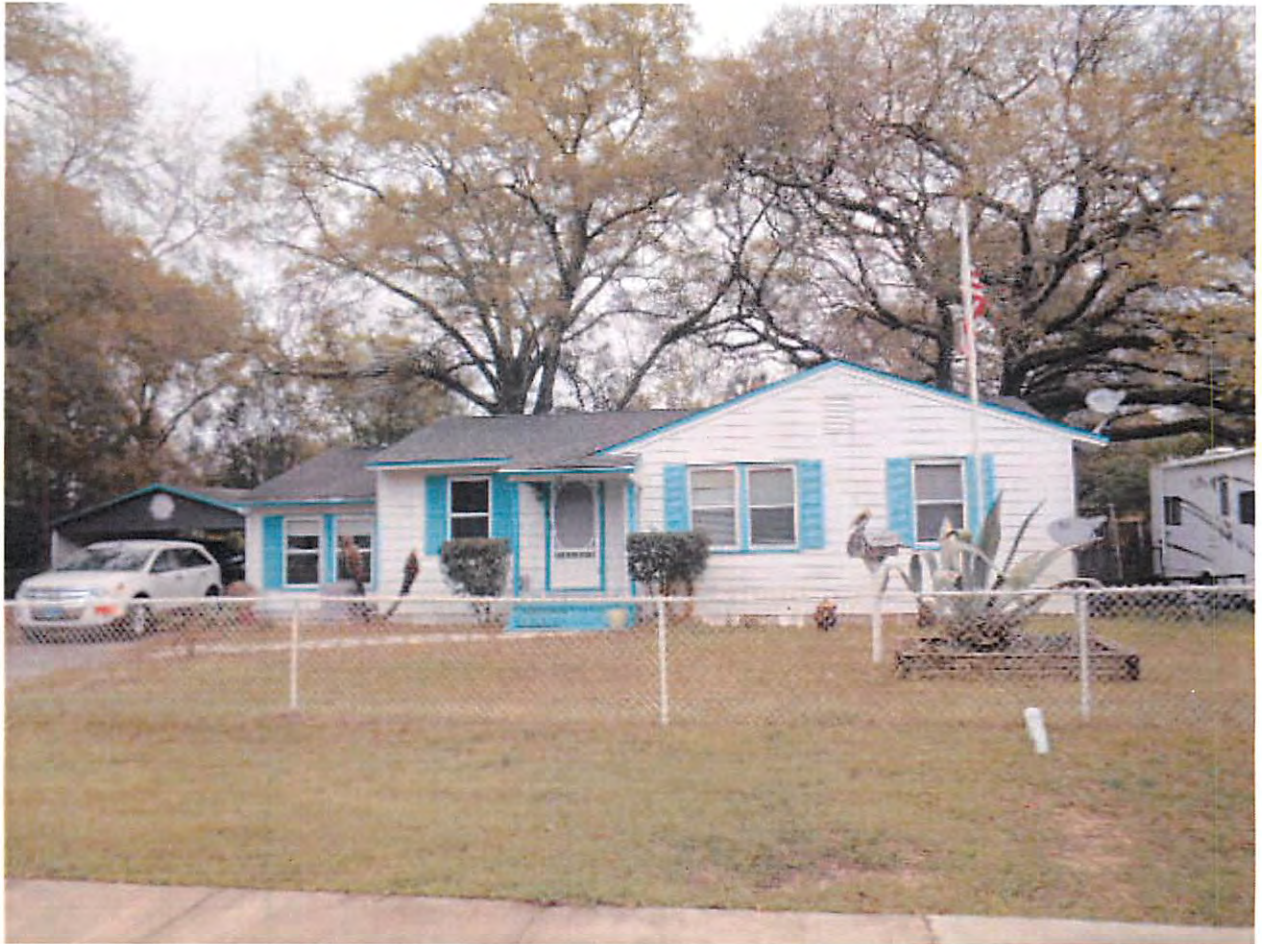
Sanitary Sewer Connection 110 Lakewood Rd – Sally Hope
