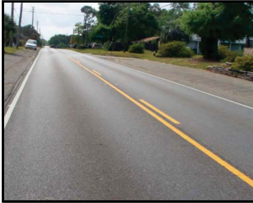
JOHNSON AVENUE: WEST
