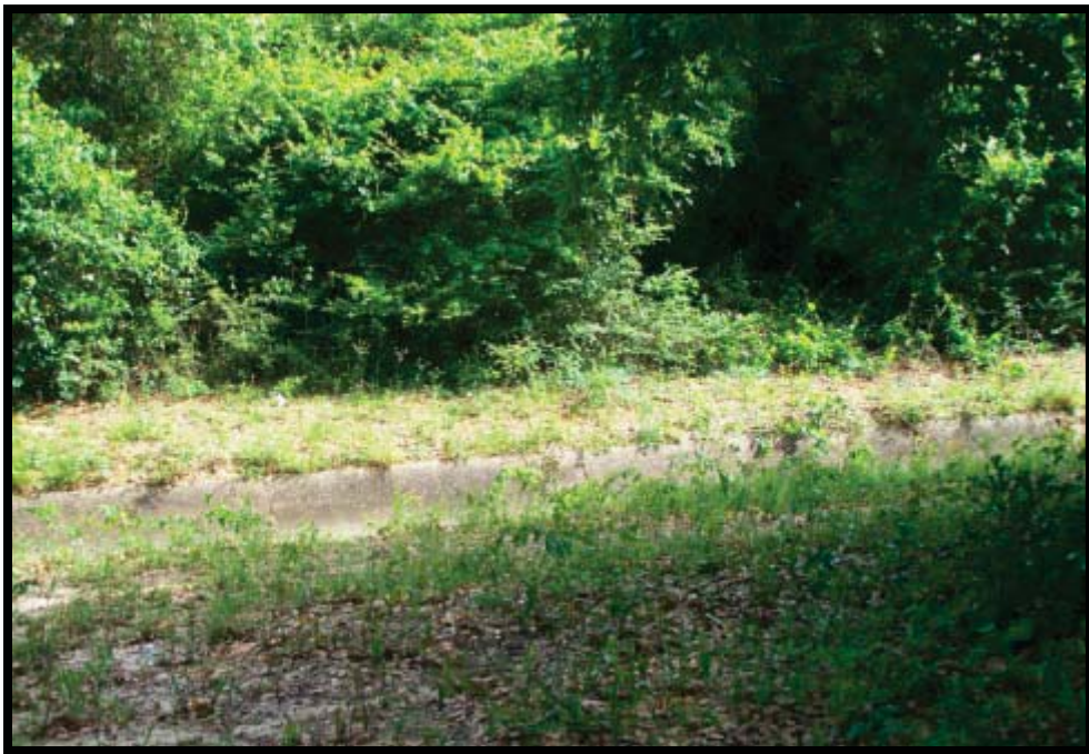
DRAINAGE AT THE REAR OF THE PROPERTY
