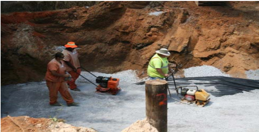
RSF “Footer” Compaction
