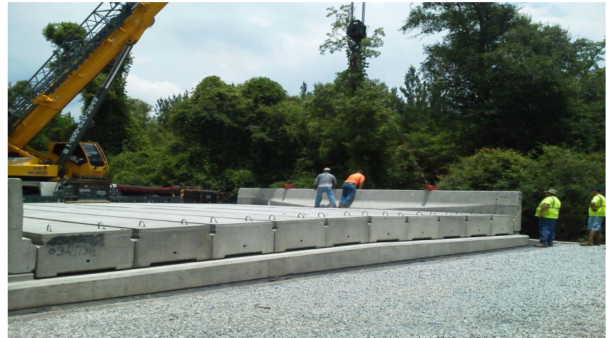
Bridge Deck Placement
