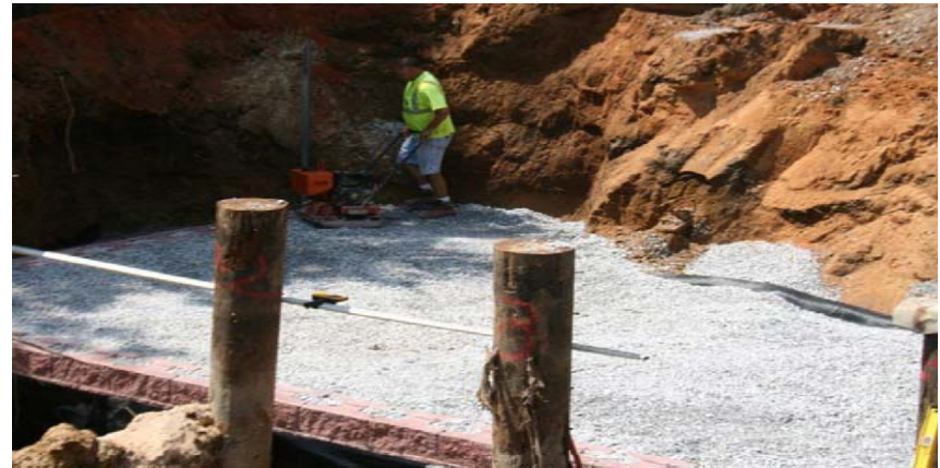
GRS Layer Compaction
