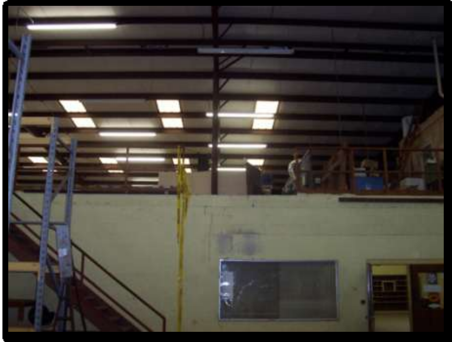
View of Mezzanine from ground floor
