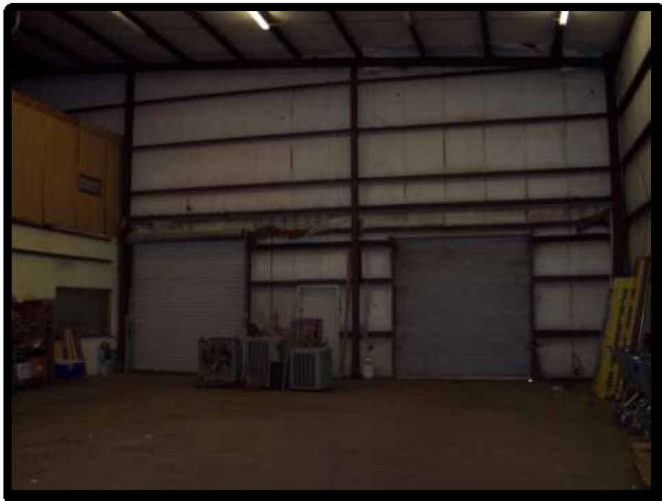
Warehouse: Two Roll Up Doors
