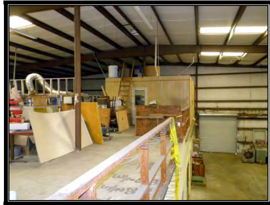
INTERIOR LOFT & SMALL OFFICE
