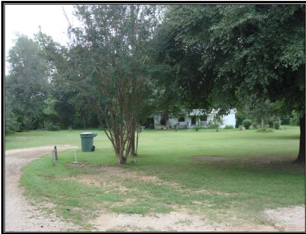
Manufactured home on subject site (not appraised) in poor condition, northern view
